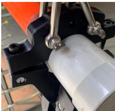
Placing Insulator on PVC Cover
