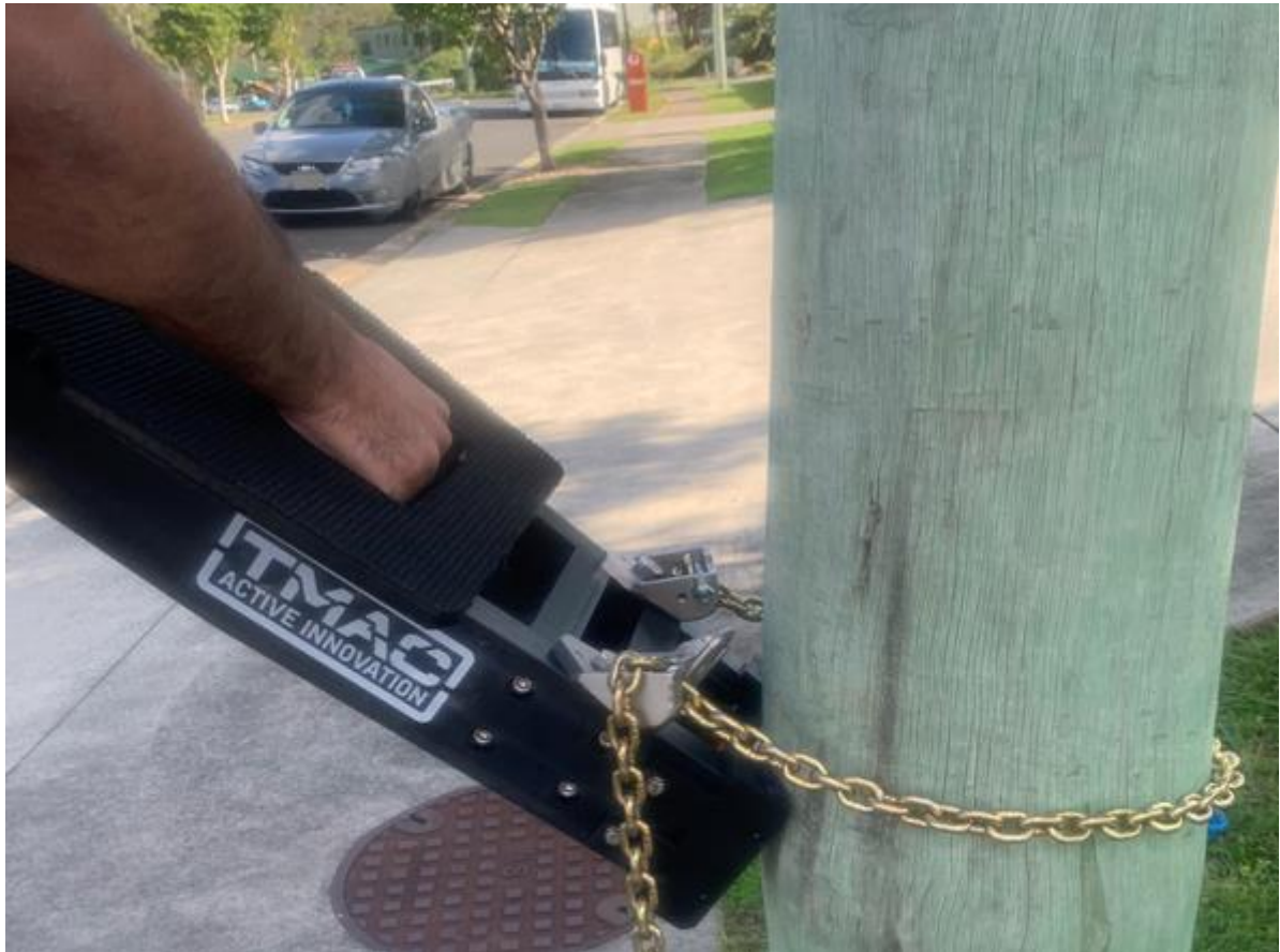
Figure 4 - Pass Chain Around Pole Tilting Platform
