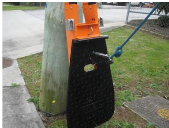
Double action snap hook through hole in the deck
