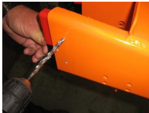
Drilling the holes for the replacement pads
